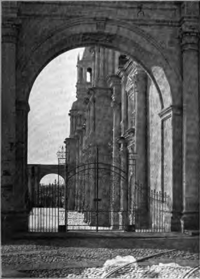
Side View of Façade, Arequipa Cathedral
